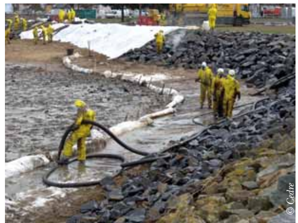
Mechanical clean-up of riprap
