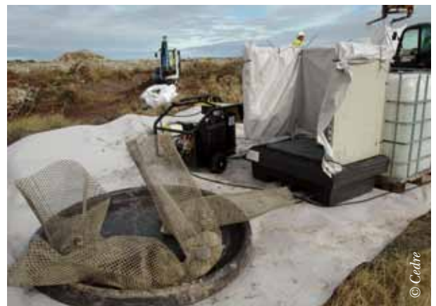
Washing pebbles on site in a booth
