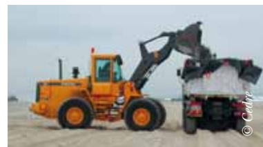
Truck and skip protected with plastic liner
