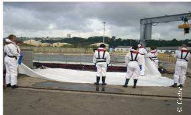
Protecting the quay with geotextile
