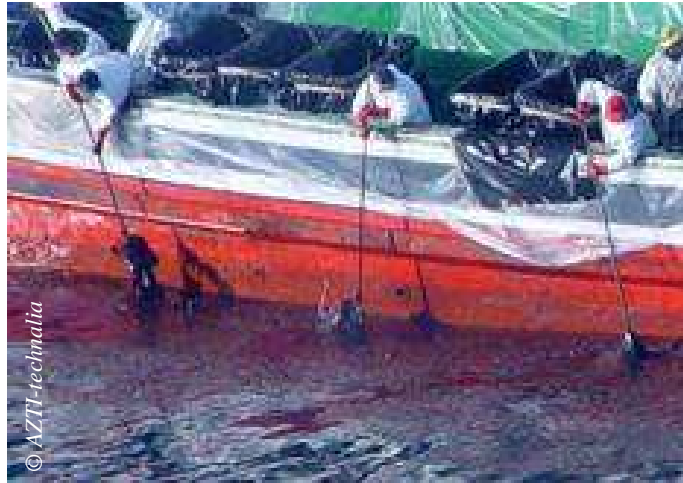
Manual recovery using adapted tools, Prestige spill, 2002
