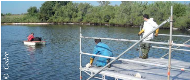
Protecting an unloading jetty
