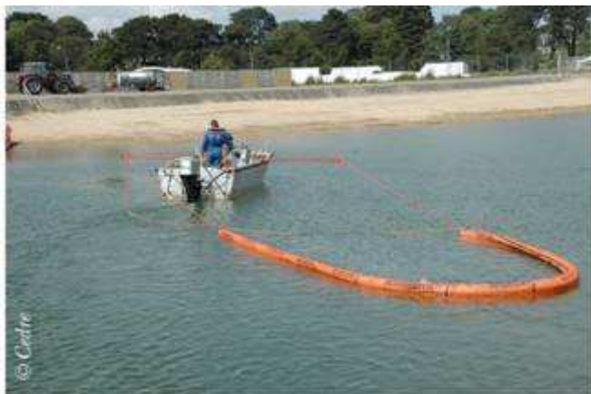
Dynamic recovery of a small spill using a sorbent boom with a ballasted skirt towed by a small boat
