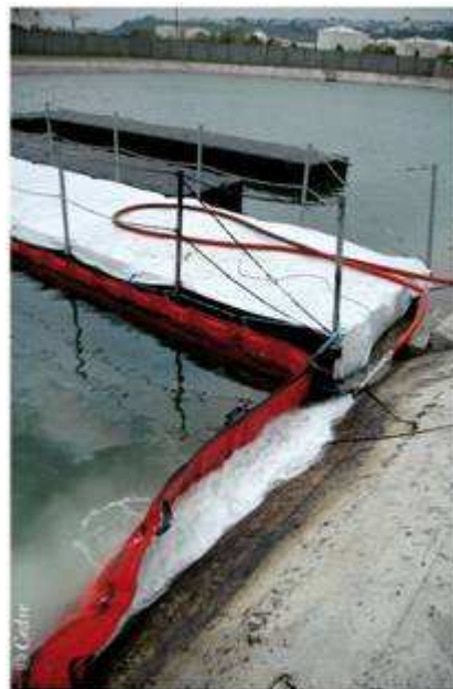
Protecting a floating pontoon using geotextile
